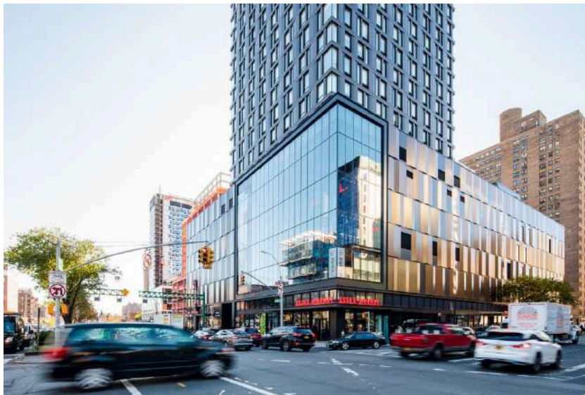
The view of the Essex from Delancey Street, with unfinished buildings behind it. Credit...Mark Wickens for The New York Times
